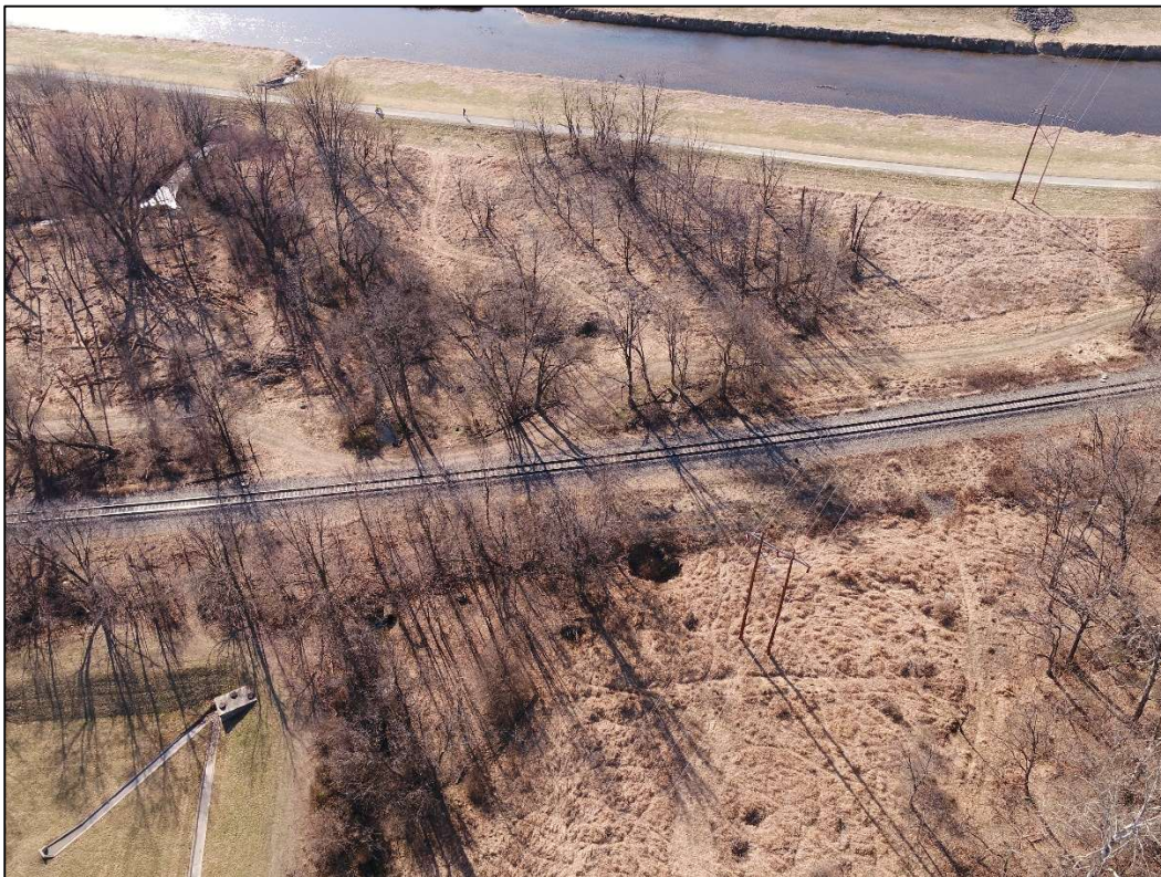
Photo 4: Photo looking west at LUA 6 and toward Codorus Creek. NP York 58, LLC stormwater basin and recent sinkhole on Sandbank Hill property is visible just east of Norfolk-Southern railroad.
